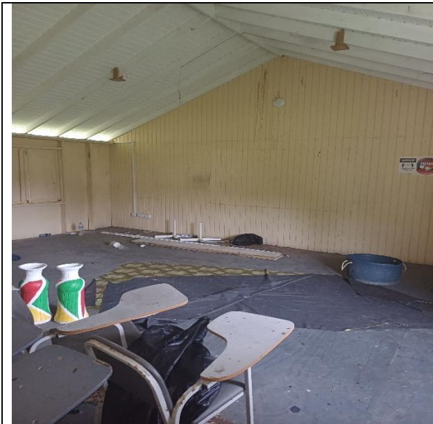
Figure 4-6: Showing internal open areas in building
