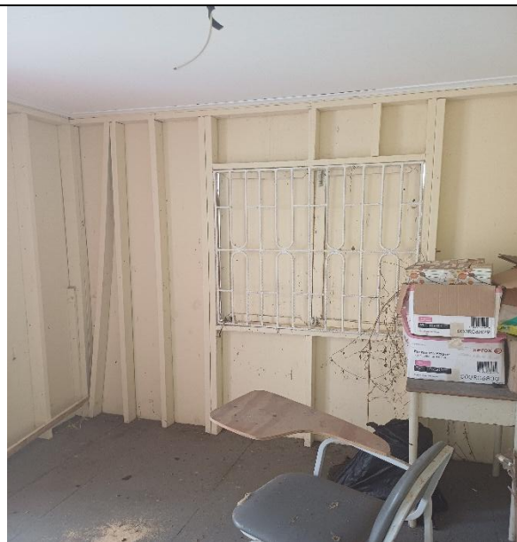
Figure 4-9: Interior space showing floor
