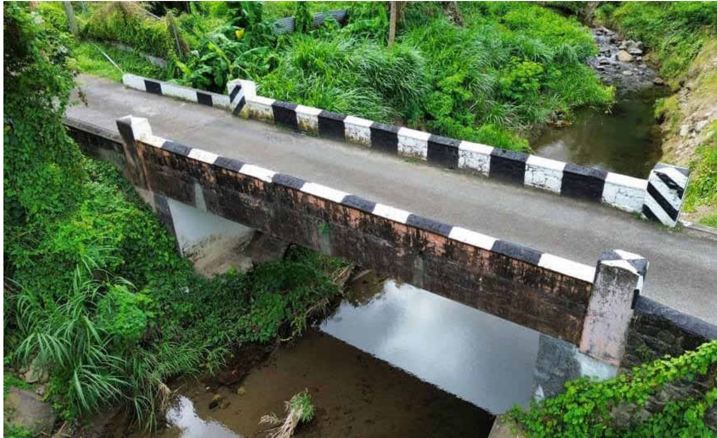
Existing Madeys Bridge – Current Condition
